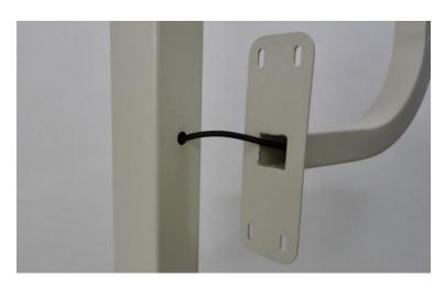
Drill a hole in the existing pole by using a Ø10 mm drill bit. To prevent rust, it is recommended to spray drilled hole with zinc spray.
