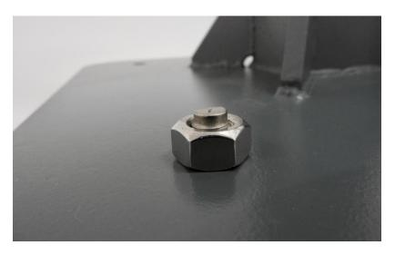
Use a spirit level to secure the right vertical position. If needed, adjust the vertical position by adding small metal plates between the metal pole plate and base. If the bolt height is 5mm or more above the nut, it is recommended to cut off the excess, as the plastic cover caps won't fit properly.
